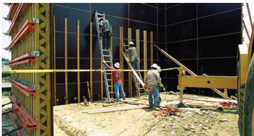
Figure 1 top: Unloading preassembled formwork.
