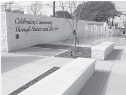
A design-build fountain sits at the pavilion's entrance, book-ended by young trees that will grow to shade concertgoers in the future.
